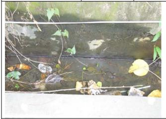
Remark 3: The general refuse in the channel should be removed and implementation of de-silting tank should be carried out (Ha Tsuen Road near RE site office)
