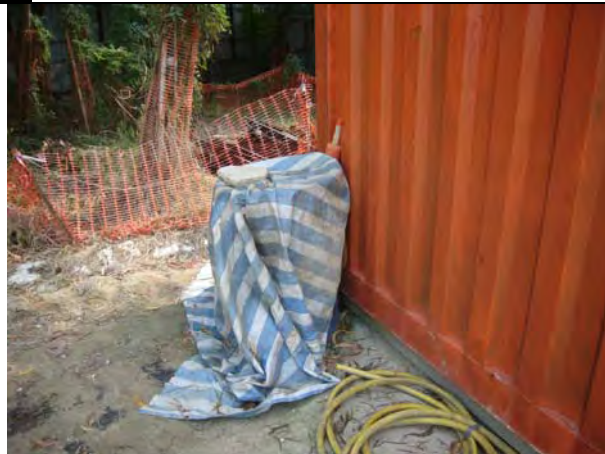
Photo 2: Free standing chemical containers without drip tray was observed at Har Tsuen PS, the contractor was reminded to provide drip tray for all chemical containers.
