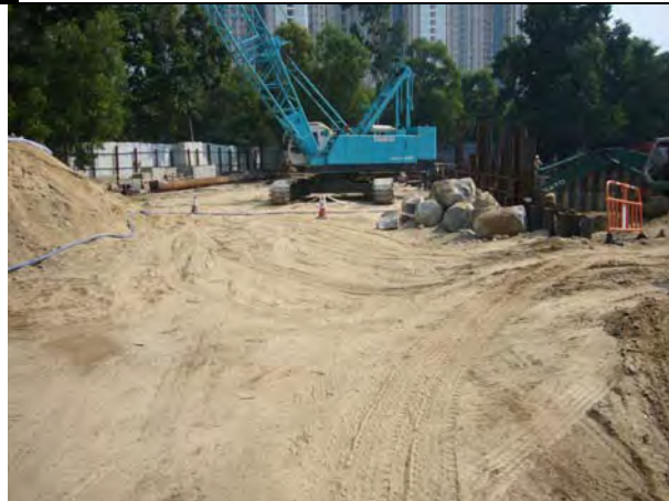
Photo 2: Dusty access road was observed at Har Tsuen PS, the contractor was reminded to provide proper dust mitigation measure to minimize dust generation.
