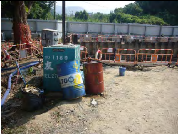
Photo 1: Free standing chemical containers without drip tray was observed at Shui Tsui San Tsuen PS, the contractor was reminded to provide drip tray for all chemical containers.
