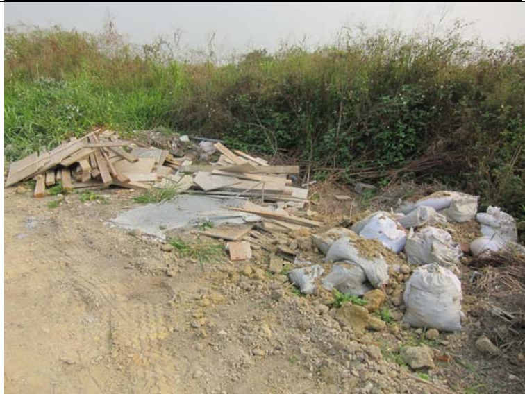
Photo 1: Scattered C&D waste was observed at Pak Sha Tsuen, Kiu Hing Road, the contractor was recommended to place the wastes in a designated location in order to keep the site tidiness.
