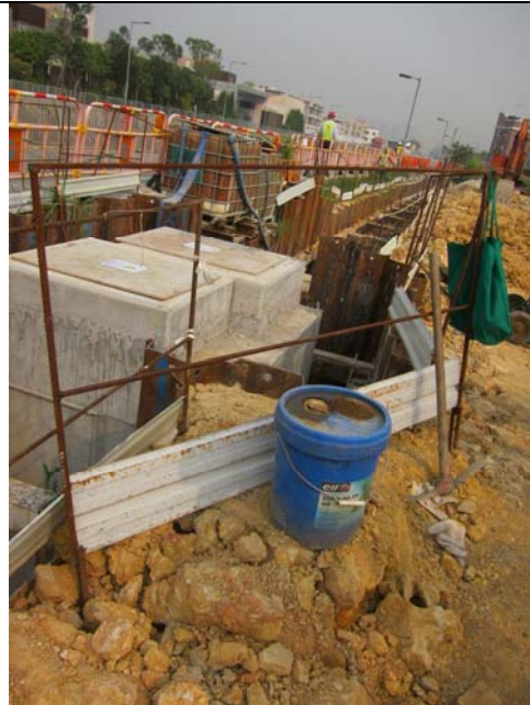
Photo 2: Free standing chemical container without drip tray was observed at Pak Sha Tsuen, Kiu Hing Road, the contractor was reminded to provide drip tray for all chemical containers.
