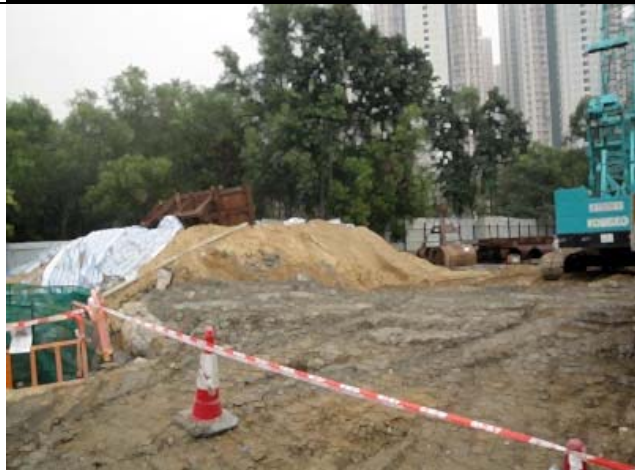
Photo 1: It was reminded that the Contractor should provide proper impermeable cover to stockpile of materials.
