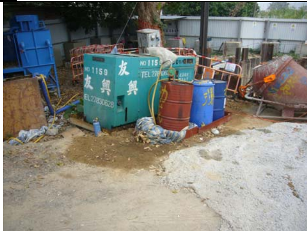
Photo 2: At Shui Tsui San Tsuen PS, although drip trays for generator and oil drums are observed, the contractor was reminded to upgrade the mitigation measures to prevent oil spillage during fueling procedures.
