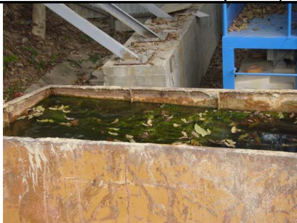
Photo 1: Sedimentation tank at Shui Tsui San Tsuen PS was full of debris, the contractor was reminded to clean to maintain the tank efficiency.
