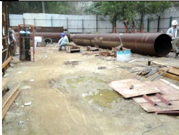
Photo 2: Accumulation of stagnant water was observed on site. The Contractor was reminded to properly clear the water.
