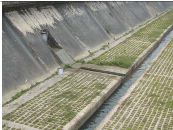
Photo 2: No Turbidity water discharged from the Tai Shiu Ha works area was observed.
