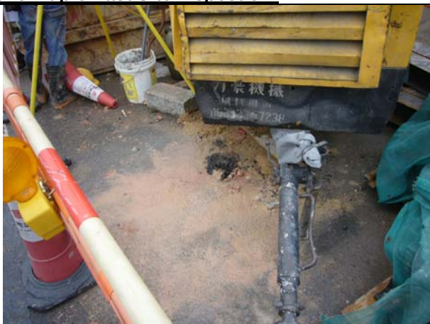
Photo 1: Oil leakage from the air compressor was observed at Tai Shiu Ha works area, the contractor was request to clean up immediately to prevent ant contamination.
