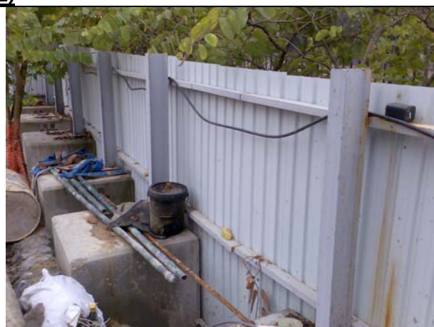
Photo 1 & 2: Free standing chemical containers without drip tray were observed Shui Tsui San Tsuen works area and Ha Tsuen PS, the contractor was requested to provide drip tray for all chemical containers.
