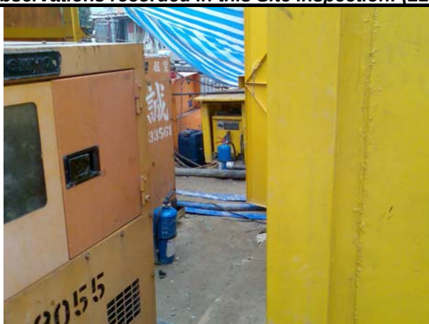
Photo 1 & 2: Free standing chemical containers without drip tray were observed Shui Tsui San Tsuen works area and Ha Tsuen PS, the contractor was requested to provide drip tray for all chemical containers.
