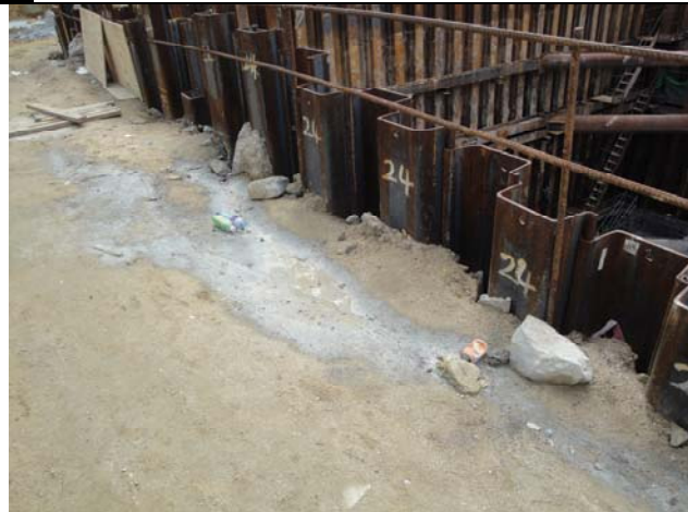
Photo 2: General refuse was found scattered around the site. The Contractor was reminded to clear the refuse in a regular basis. (HSPS)
