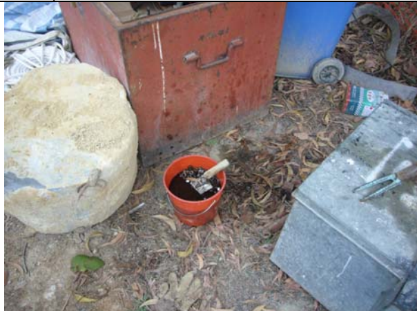
Photo 4: Free standing chemical container without drip tray was observed, the contractor was reminded to provide drip tray for all chemical container in the site area.
