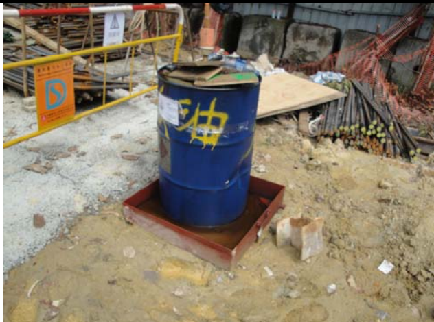
Photo1: The Contractor was reminded to remove the C&D waste on the chemical container and to regularly clear the water accumulated within the drip tray. (HSPS)
