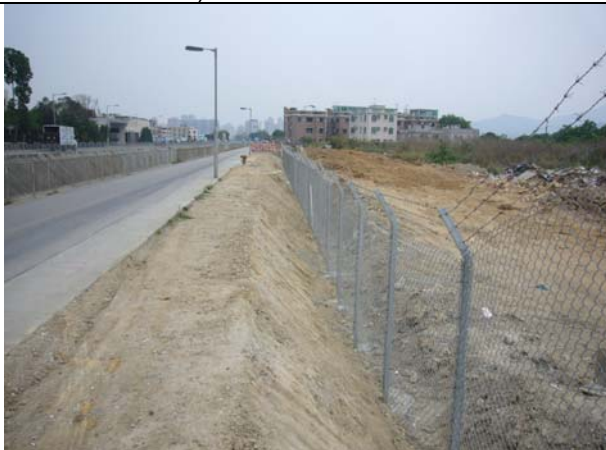
Photo3: Stockpile without cover was observed at Kiu Hing Road, the contractor was reminded to provide proper mitigation measure to prevent dust generation.
