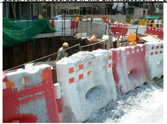
Remark 1: Some spillage of concrete was observed on plastic road barriers. The Contractor was reminded to regularly clean the site area after concreting works.
