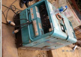
Generator without drip tray was observed. Drip tray or removal of the equipment from the site is required
