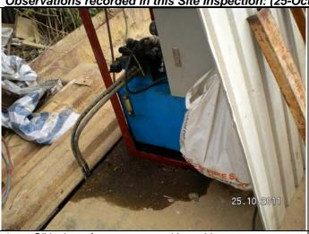
Oil leakage from generator without drip tray was observed in the Ha Tsuen Rd construction site. Clearance of the oil and Drip tray or removal of the equipment from the site is required.
