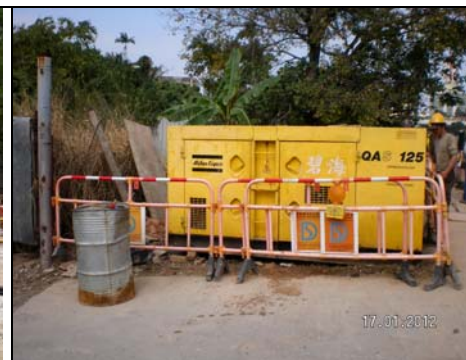
Photo 2: Oil drum without drip tray at Tai Shu Ha Tsuen.
