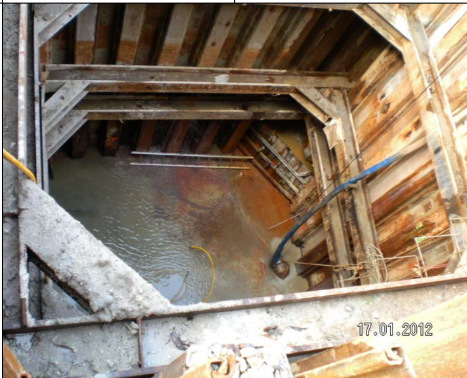
Photo 3 Groundwater pumping at Ha Tsuen Pumping Station.
