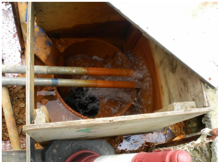
Photo 1 Discharge of groundwater at Ha Tsuen Pumping Station
