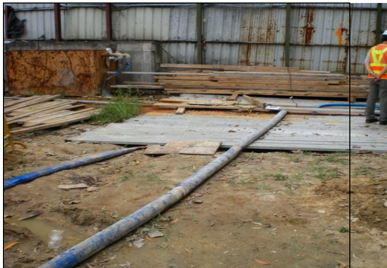
Photo 2 Sedimentation of site discharge
