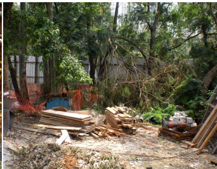
Photo 4: Fallen tree/branches at Ha Tsuen Pumping Station
