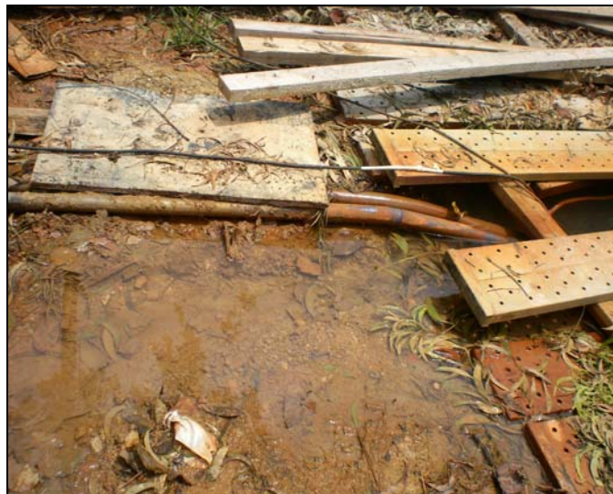
Photo 2: Flooded area at Ha Tsuen Pumping Station
