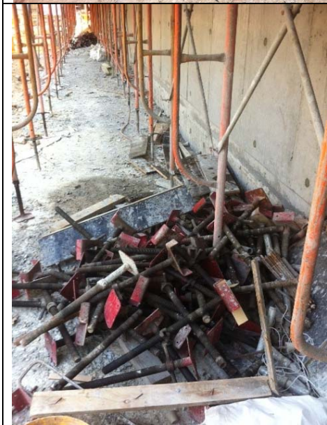
Photo 2 and 3: Scattered of C&D waste was observed Ha Tseun Sewage Pumping Station, housekeeping should be improved.
