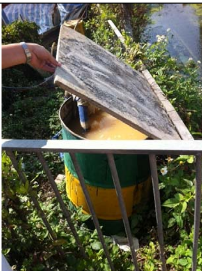
Photo 1: The de-silting tank in the working area of Sham Chung should be cleaned regularly in order to maintain the de-silting capability.
