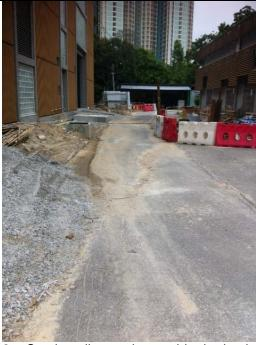
Sandy trail was observed in the haul road of Ha Tsuen Sewage Pumping Station, the Contractor should sweep the sandy trail and apply water spray regularly to minimize fugitive dust.
