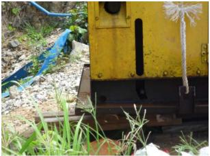
Stagnant water inside the drip tray of a generator was observed at Sham Chung Works Area, the Contractor should drain the water away as a mosquito control.
