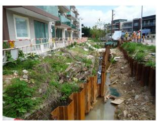
Oil stain was observed in the stagnant water in Sham Chung Works Area, the Contractor should remove the stagnant water with proper treatment.
