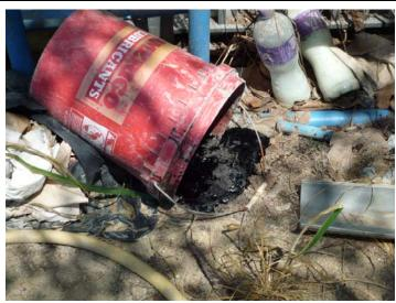
Chemical spilling was observed in the Ha Tsuen Sewage Pumping Station, the Contractor should remove the chemical container in chemical storage area and clean the chemical spill with proper approach.
