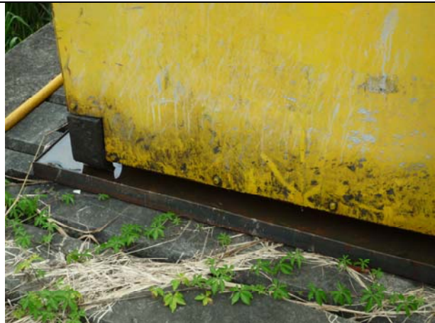
Photo 1: Stagnant water was observed in the drip tray in Sham Chung Works Area, the Contractor should clean the stagnant water regularly to prevent mosquito breeding.
