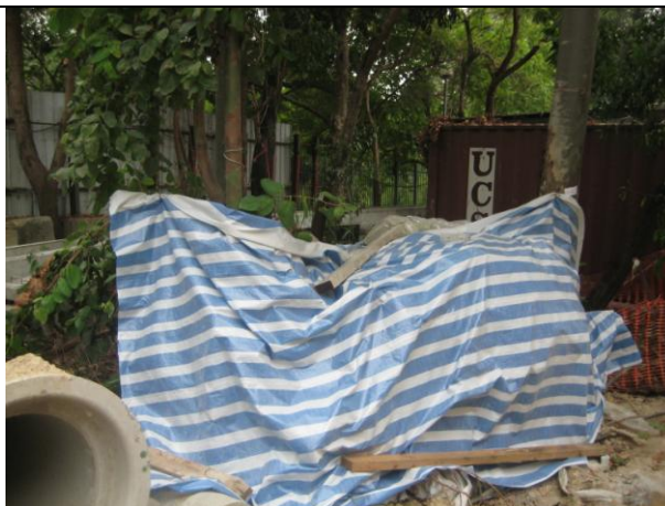
Photo 2: Construction materials were found underneath the protected trees at Ha Tsuen Sewage Pumping Station. The Contractor was reminded not to store materials underneath the trees.
