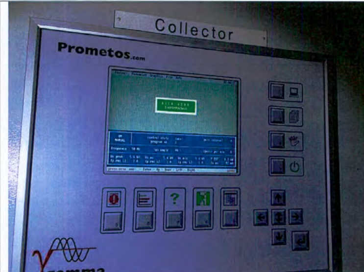
Typical mode setting for 40% ignition angle and check voltage and current of ESP Collector unit on screen after 30 minutes.
