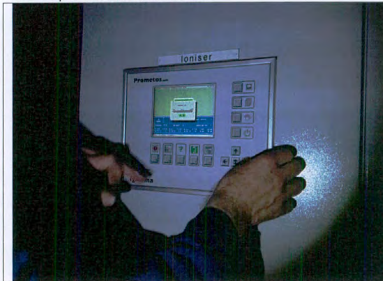
View on typical manual mode setting of HV output of ESP Ioniser by adjusting ignition angle on screen
