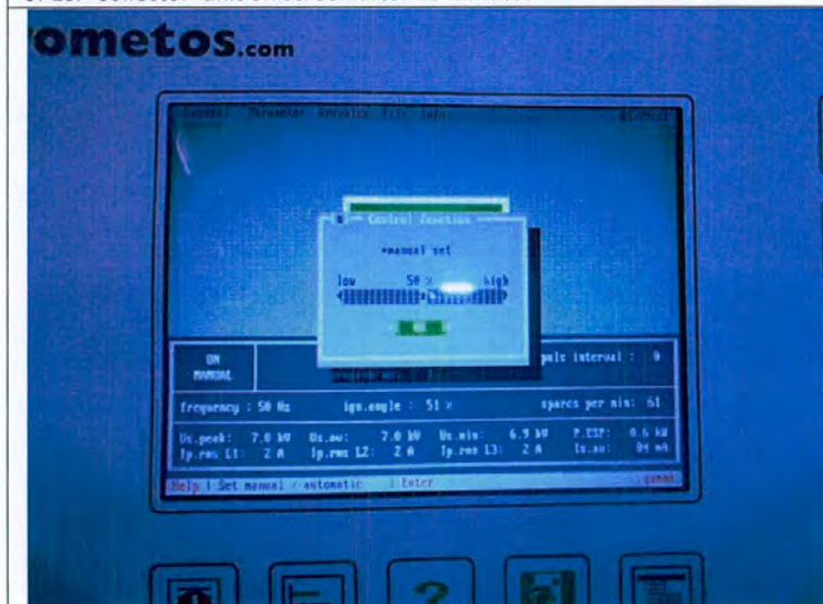
Typical manual mode setting for 50% ignition angle and check voltage and current of ESP Collector unit on screen after 30 minutes.
