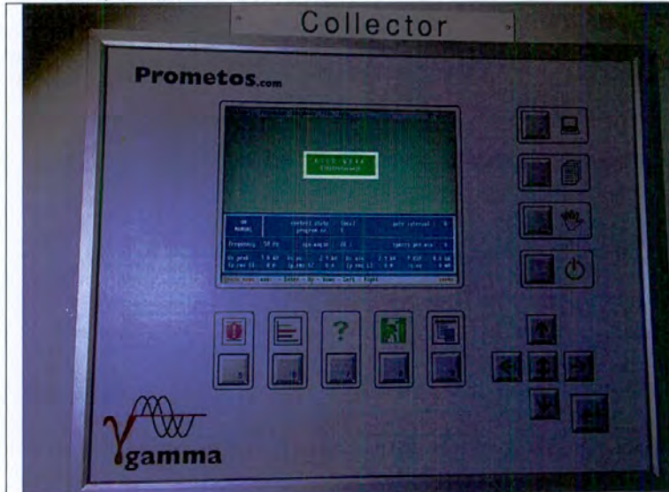
Typical manual mode setting for 20% ignition angle and check voltage and current of ESP Collector unit on screen after 20 minutes.
