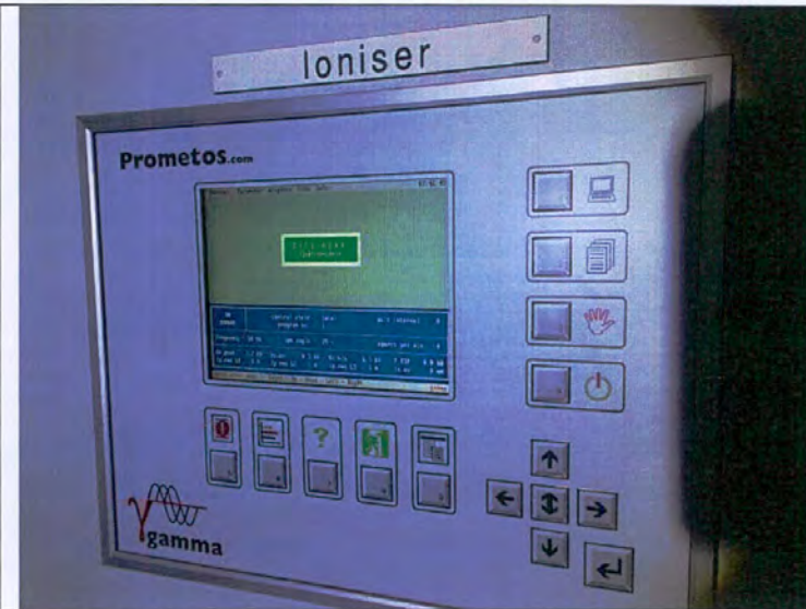
Typical manual mode setting for 20% ignition angle and check voltage and current of ESP Ioniser unit on screen after 20 minutes.
