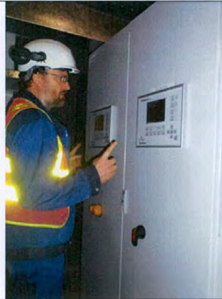
View on energizing of HV control panel (Ionizer) in auxiliary plant room in B2 of EVB
