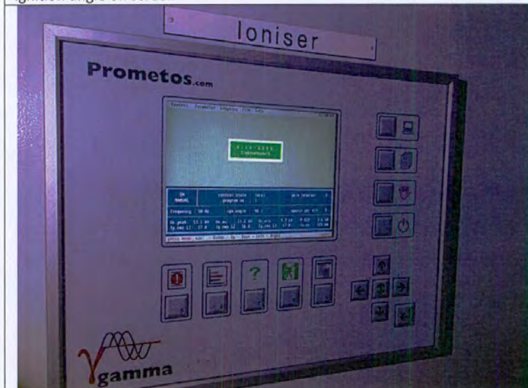
Typical manual mode setting for 40% ignition angle and check voltage and current of ESP Ioniser unit on screen after 30 minutes.
