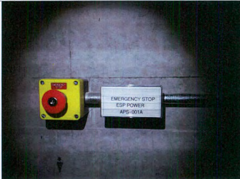
View on typical emergency stop installed at entrance of ESP area A, B & C with identification label (APS-001A)
