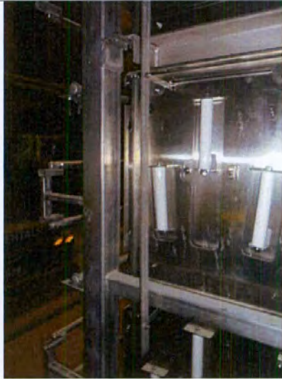
End view on typical common earth tape connected with ESP modules on rack at APS plant room in B2 of EVB
