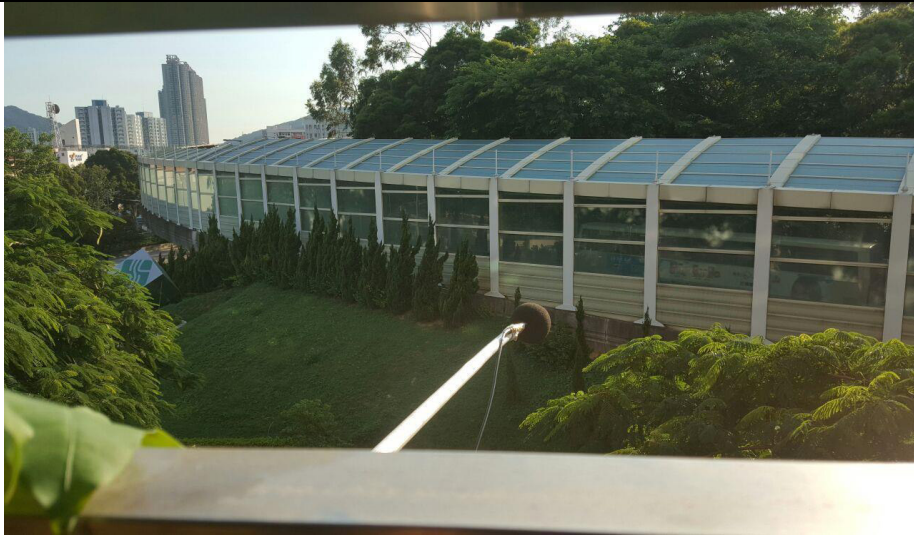
N6 - Scenery Court, Podium near Block 1 - 4/F
