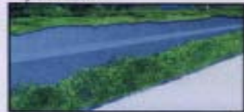
OPTION: Drainage channel with grassing along edge
