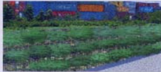
Drainage channel showing planting in channel edge
