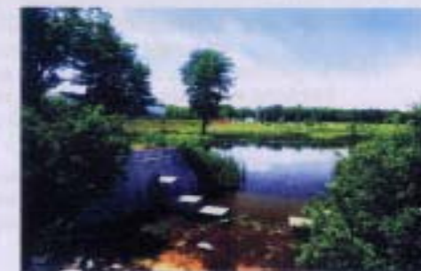
Weir construction at specific locations.
