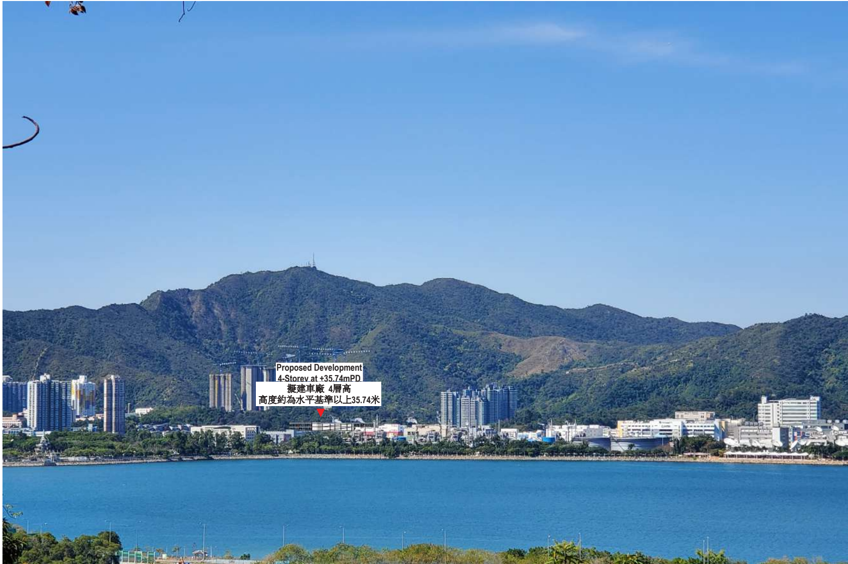
VP6: From Tai Po Road across the Tolo Harbour (Approx. 3km from site)
