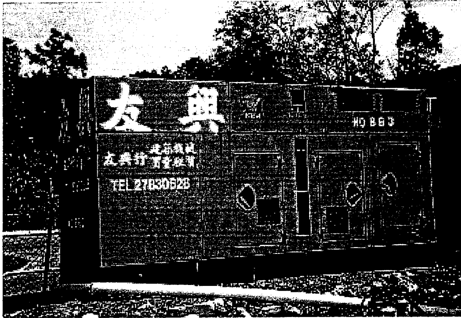
Generator, super silenced, 70 dB(A) at 7 m.
