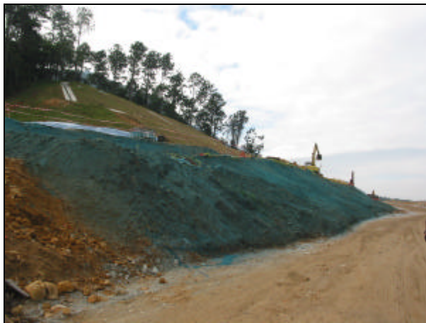
Figure 6-1 – The temporary slope near Monte Vista.
