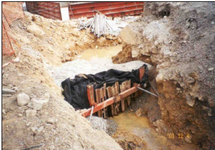
Figure 6-5 The high S.S. runoff was filtrated by broken rock.
