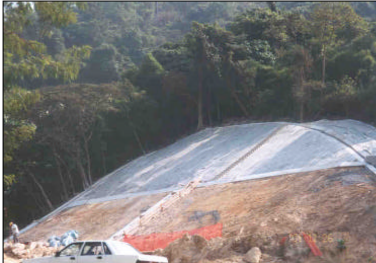
Figure 6-6 The hydroseeded slopes near entrance No. 6
