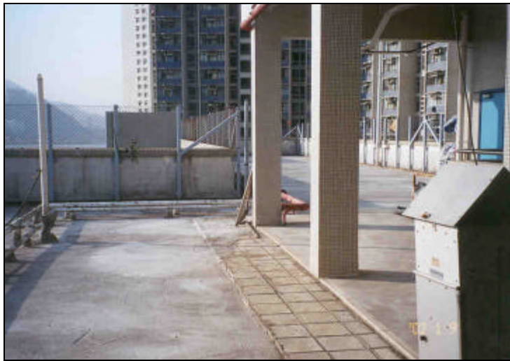
Figure 6-7 Roof waterproofing works at Ma On Shan Lutheran Primary School.
