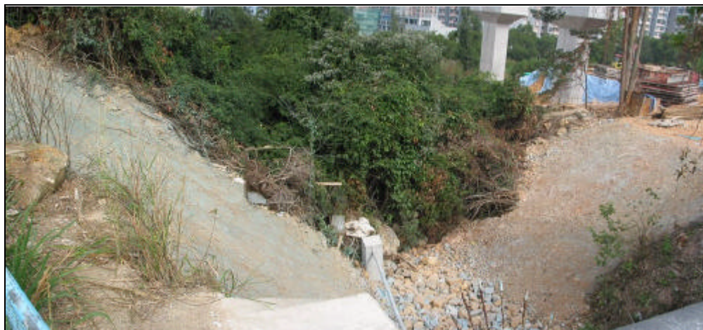
Figure 6-2 – The hydroseeded slope at the upstream of discharge point no.5.
