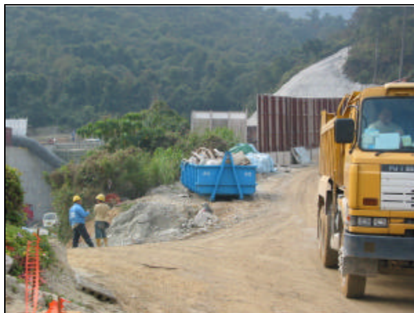
Figure 6-1 – The rubbish tray at Portal D area.
