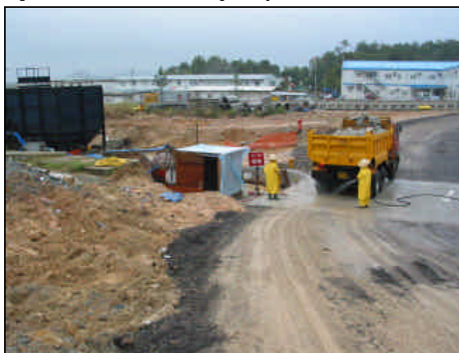
Figure 6-1 – The wheel washing facility at new access.
