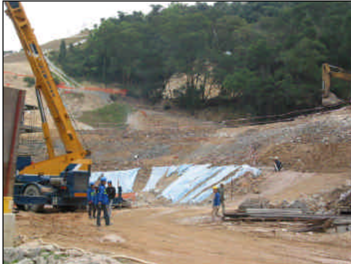
Figure 6-3 – The water sprayers and covered slope between Lee On Estate and Monte Vista.
