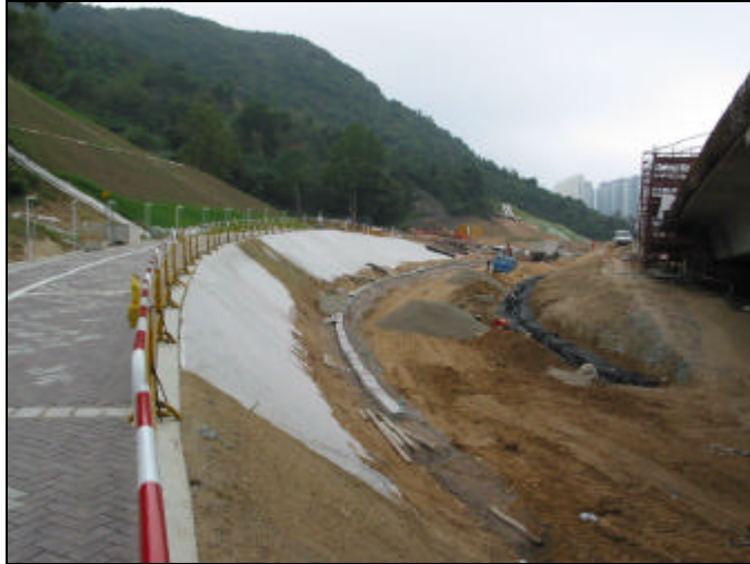
Figure 6-3 – The hydroseeded slope near TA bridge.
