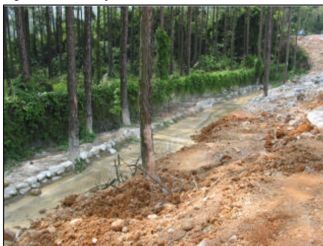
Figure 6-1 – The silty channel near Portal D.
