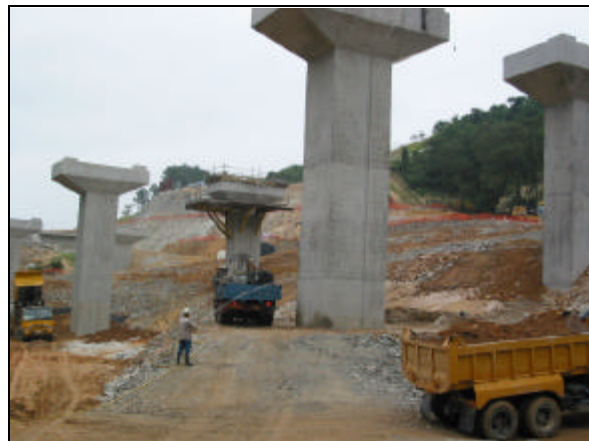
Figure 6-4 - Water sprayers are operating at backfilling slope.
