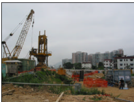
Figure 6-7 - The bore piling machine and sedimentation tanks at TD bridge area
