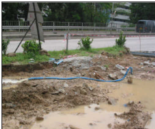
Figure 6-6 - The direct discharge runoff from the site
