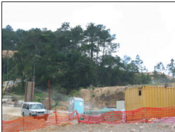
Figure 6-3 – Water sprayers are operating at Portal D area.
