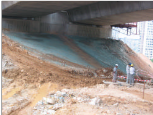
Figure 6-5 – The hydroseeded slope under TB bridge.
