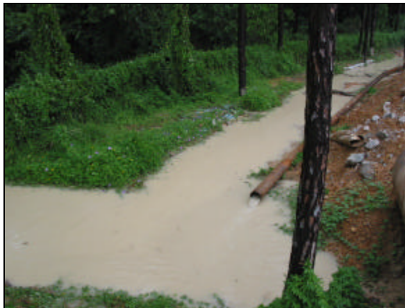
Figure 6-1 – The silty channel near Portal D area.
