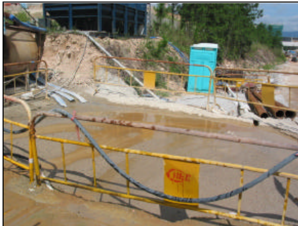
Figure 6-5 - The desilting pit at site access near Cheung Muk Tau Village
