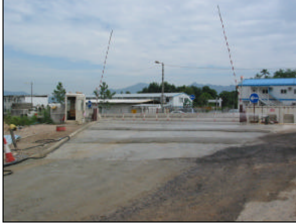
Figure 6-4 – The bunds were installed before the new access.
