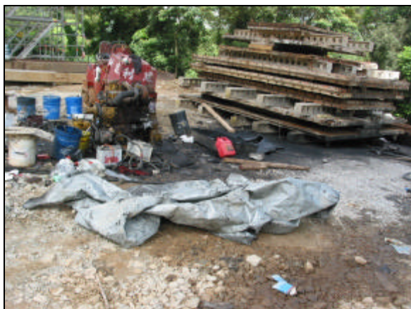
Figure 6-3 – The workshop under TC bridge.
