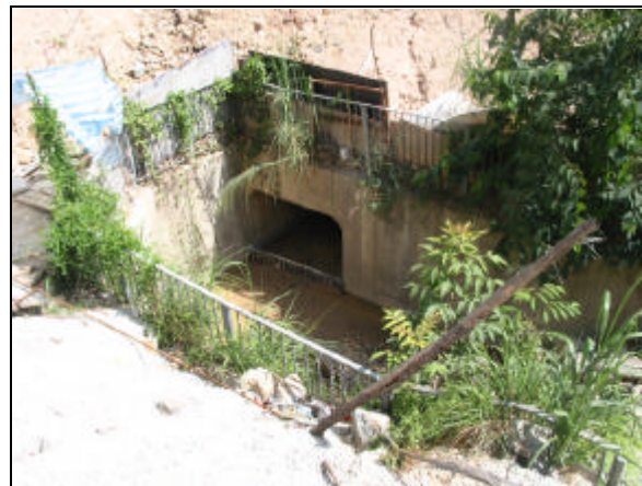
Figure 6-2 - The silty channel at discharge point no. 7
