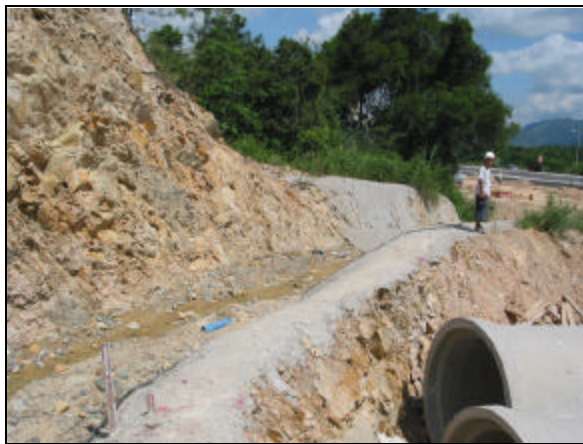
Figure 6-1 – The silty channel near Portal D area.
