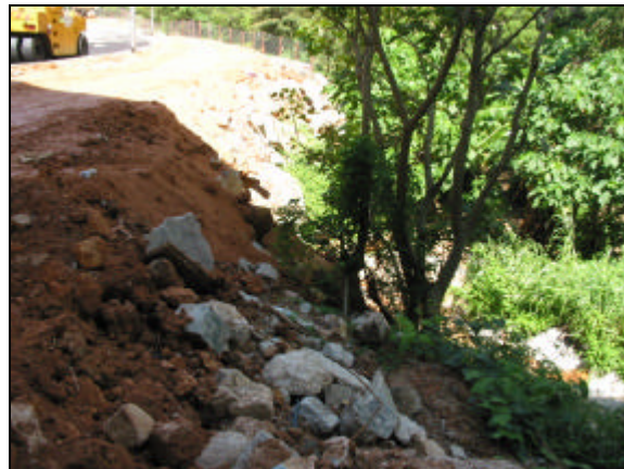
Figure 6-7 - The exposed surround of channels near discharge point no.3
