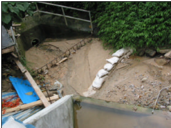
Figure 6-1 – The silty channel at stream S28.
