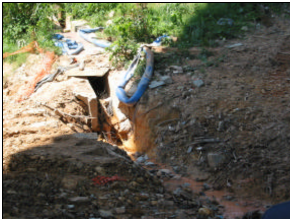
Figure 6-6 - The exposed surround of channels near discharge point no.4
