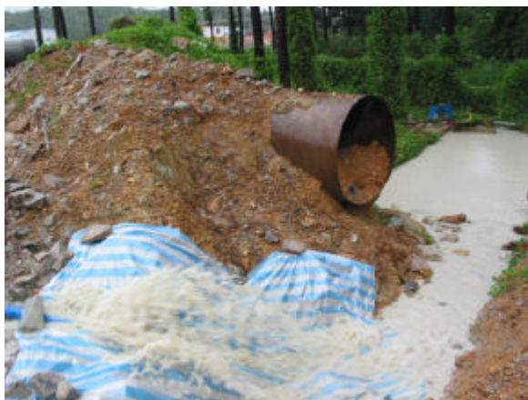
Figure 6-1 - Surface runoff near discharge point no. 8 after rainstorm
