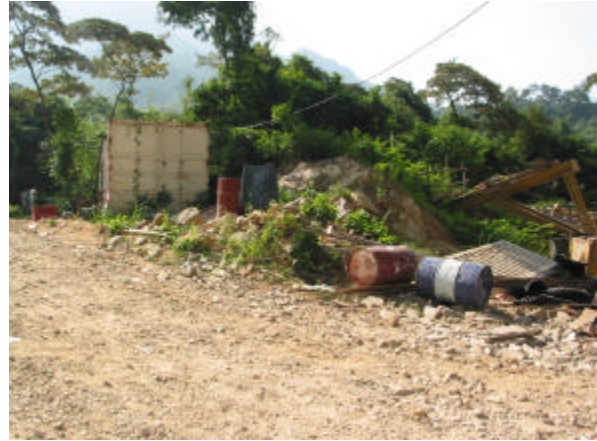
Figure 6-6 - Poor housekeeping under Bridge C.
