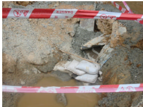
Figure 6-2 - Sand trap near discharge point no. 3
