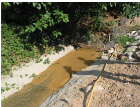
Figure 6-2 - Sand trap near discharge point no. 6
