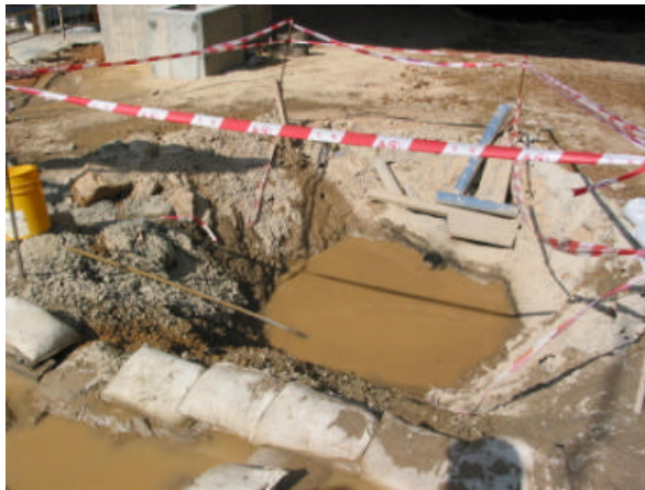
Figure 6-3 - Sand trap near Discharge Point 3.
