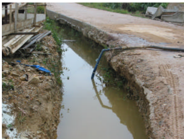
Figure 6-1 - Drainage channel S2A.
