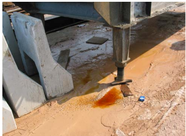
Figure 6-2 – Oil leakage at Gate 10 Storage Yard.
