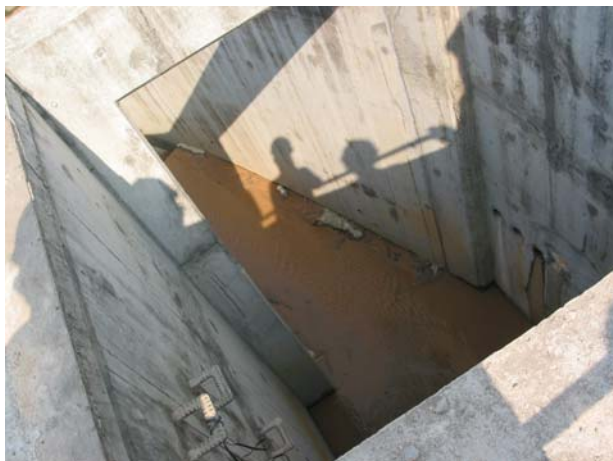
Figure 6-1 – De-silting pit at Discharge Point 3.
