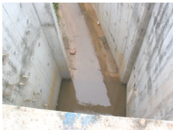
Figure 6-1 - De-silting pit at Discharge Point 3
