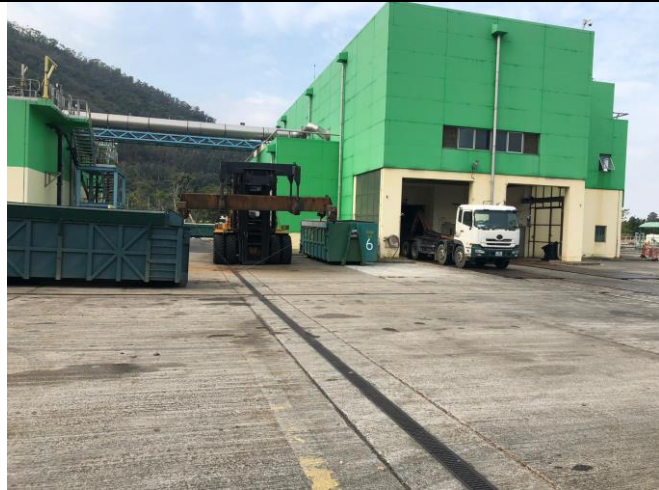
Sludge Dewatering House
