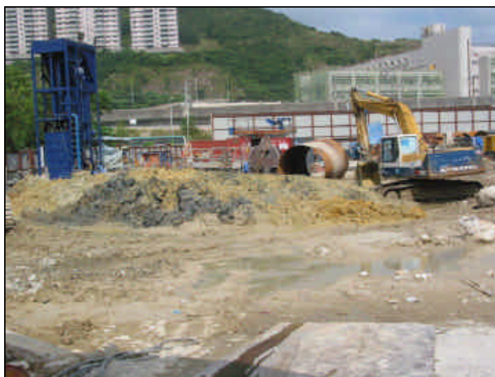
Figure 6-1 The stockpile of the excavated material
