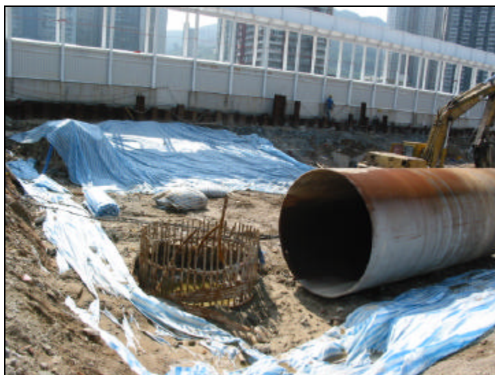
Figure 6-1 The covered slope of pile-cap
