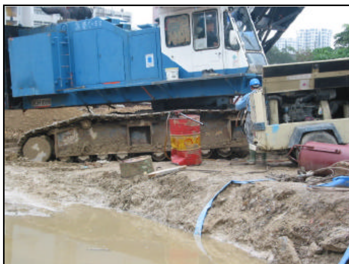
Figure 6-1 The diesel drum without drip tray
