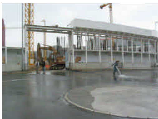
Figure 6-1 The wheel washing at site access
