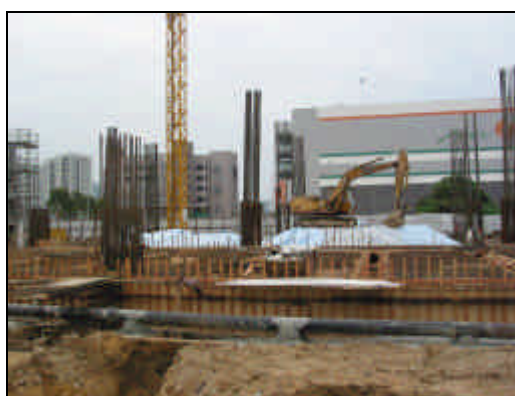
Figure 6-2 The covered stockpile
