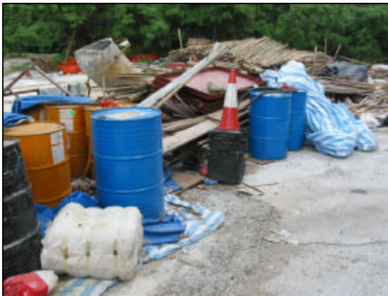
Figure 6-3 Oil drums without drip tray
