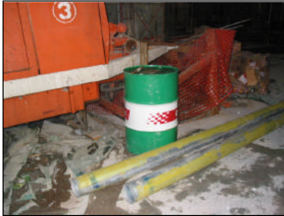
Figure 6-2 Oil drums without drip tray
