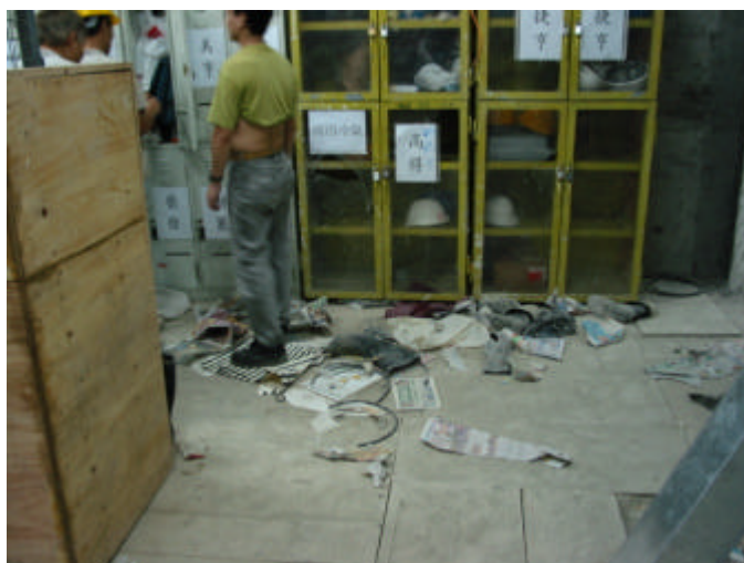
Figure 6-1 General refuse accumulating on 3/F.
