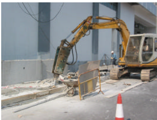
Figure 6-1 Dust generated from earth breaking operation.
