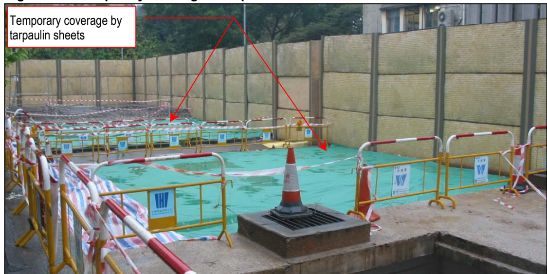
Figure 5-1 Temporary coverage of unpaved area
