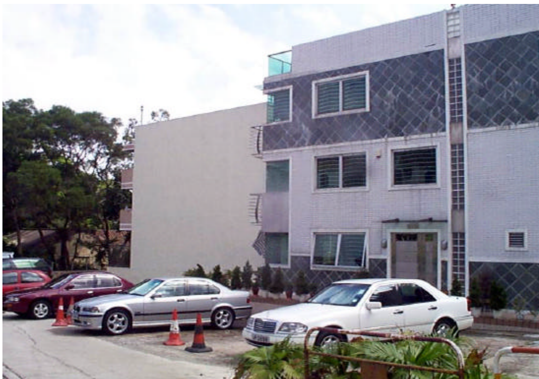
Monitoring Point CNM 1 – Wu Kwai Sha New Village
