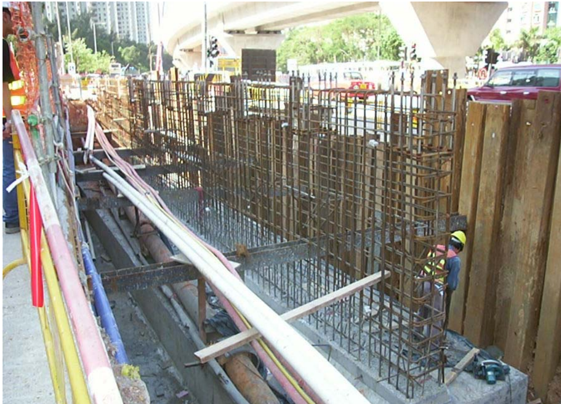
Date: 13 November 2003 Location: Near Kam Lung Court
