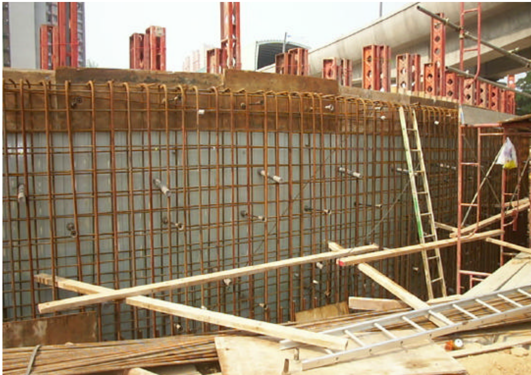
Date: 5 March 2004 Works: Retaining Wall Construction Location: Near Lee Wing House
